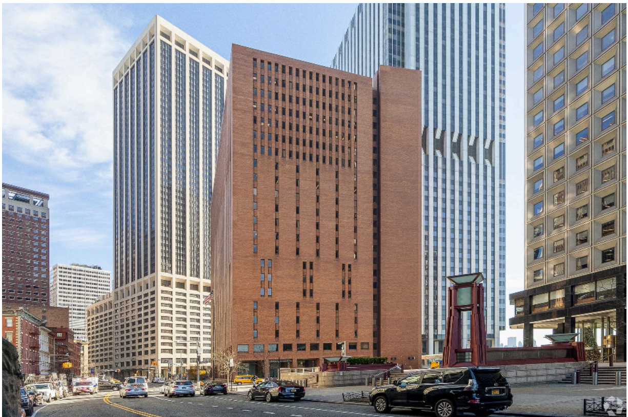
Exterior brick on the former 25 Water St. tower was replaced or covered with a new facade. (CoStar)
