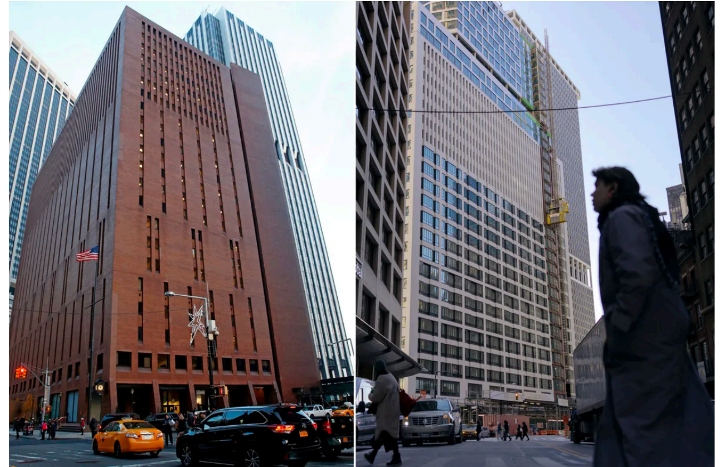
25 Water St., before and after renovation. Source: AP Photo; Bloomberg
